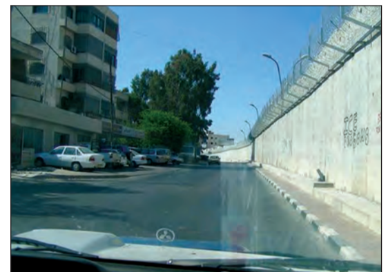
Part of the 'security wall'
